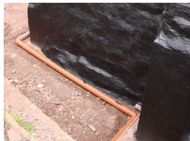
Triton TT Vapour Membrane to external walls
